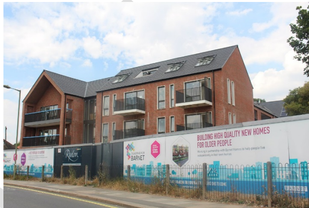
Ansell Court under construction
