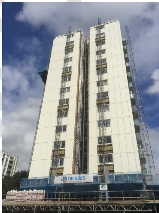
Cladding replacement works underway at Granville Road
